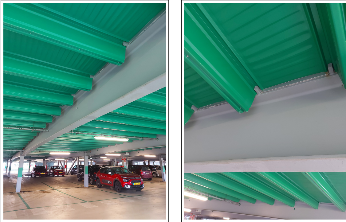
Figure B.10: an example of carpark application of the IPE550A solution. Sheeting is not fixed with welded wings in this configuration: bars welded on the top flange are used for supports.
